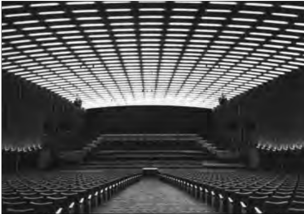
Fig. 9.11 Luminous ceiling of the broadcasting studio of the Hesse Radio in the year 1956: the lighting installation qualifies as “completely glare-free” by the standards of the time. (Rick-Lenze et al,1987)
